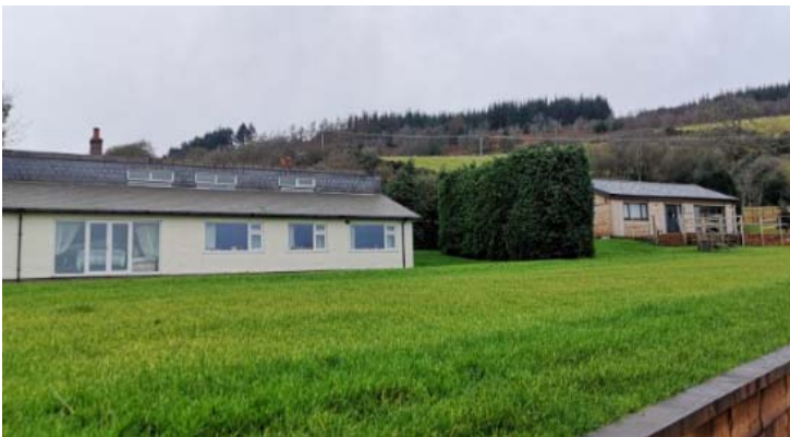
Main dwelling to the left with ancillary building screened off
