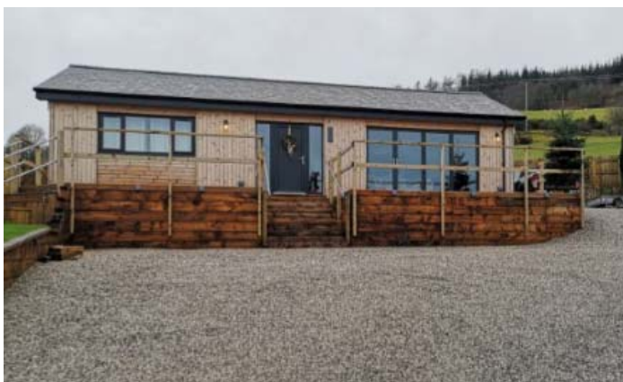
Existing ancillary building frontage
